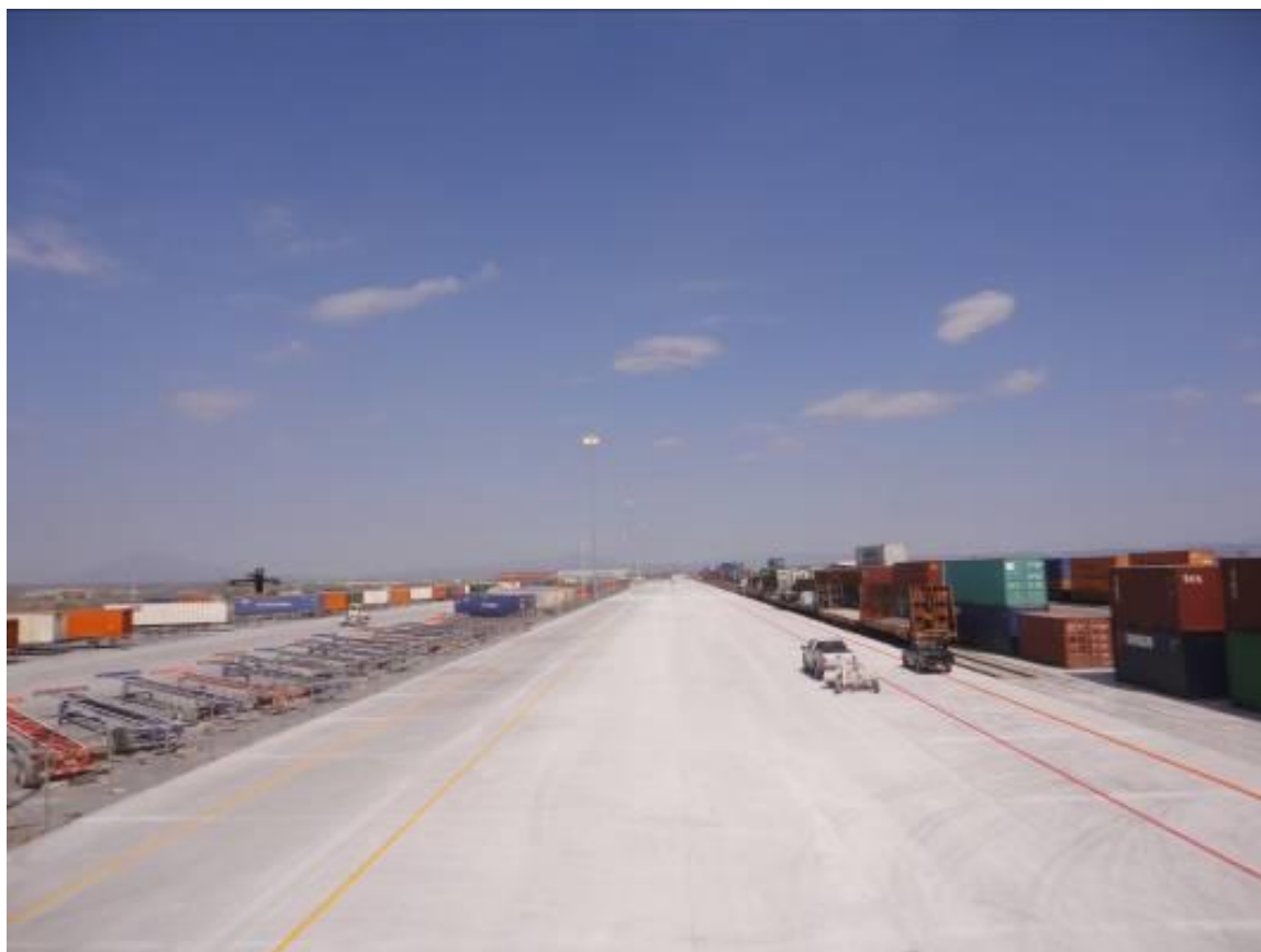
KCSM. Terminal intermodal en Salinas Victoria N.L.
