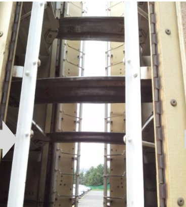
4. Bridge plates to connect railcars while loading
